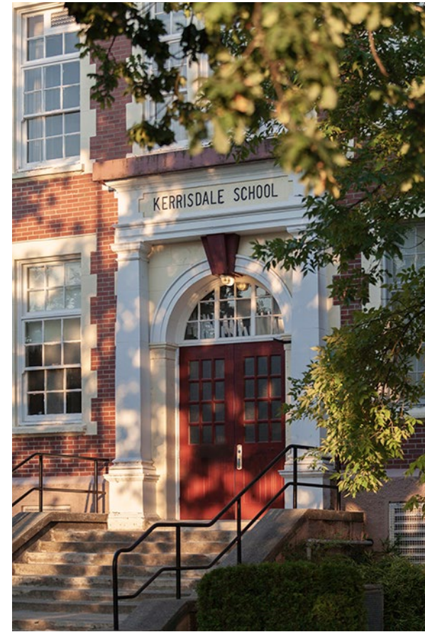
KERRISDALE ELEMENTARY SCHOOL
